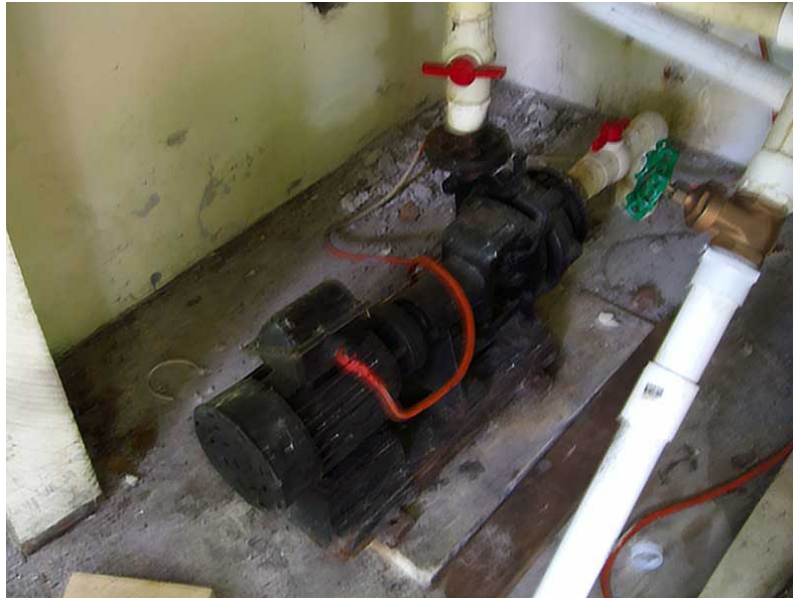
Pictured above is the Current three phase 5 hp motor pump used on Matamanoa island resort located in Fiji.
