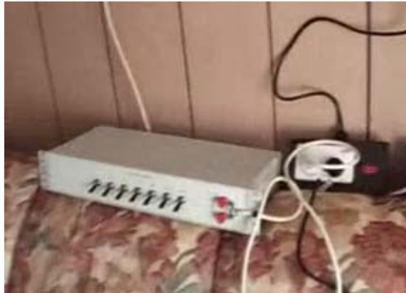
Tuning binary cap bank connected to the air con and mains
