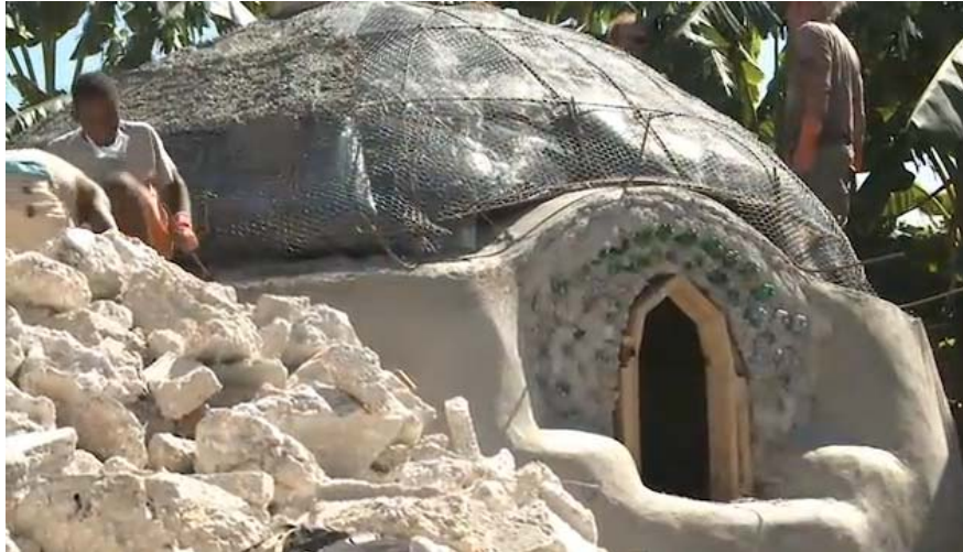
Earthquake proof dome - Earthship Haiti educational rebuild project
